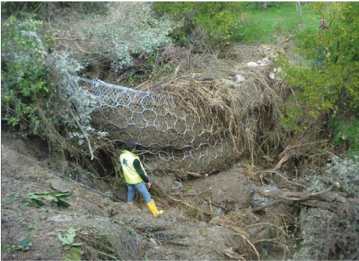
Filled and overflowed debris flow protection net.
