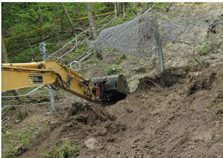
Emptying of a hillslope debris flow protection net from the downslope side using an excavator.
