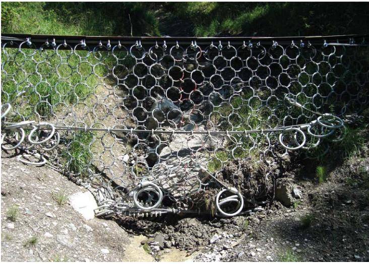
Congestion of the basal opening due to partial filling of a debris flow protection net.
