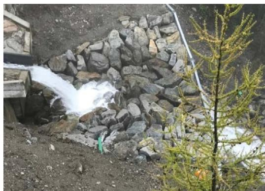
Pre-filled barrier using large blocks, seen from above (Image: [I]).
