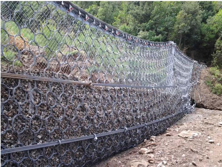
Debris flow protection net filled by bedload transport.
