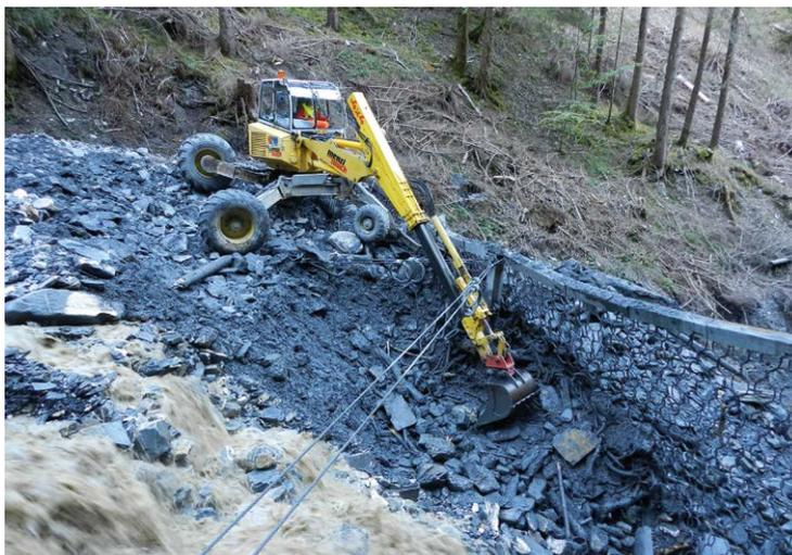
Emptying of a debris flow protection net from the uphill side using a walking excavator.
